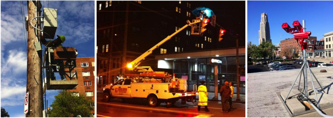
Figure 1: Deployment of cameras and edge computers to the Craig Street and Fifth Avenue intersection in Pittsburgh, PA. Eight cameras were mounted on traffic signal poles. The cabinet containing the computers and other equipment were mounted on a nearby utility pole.
