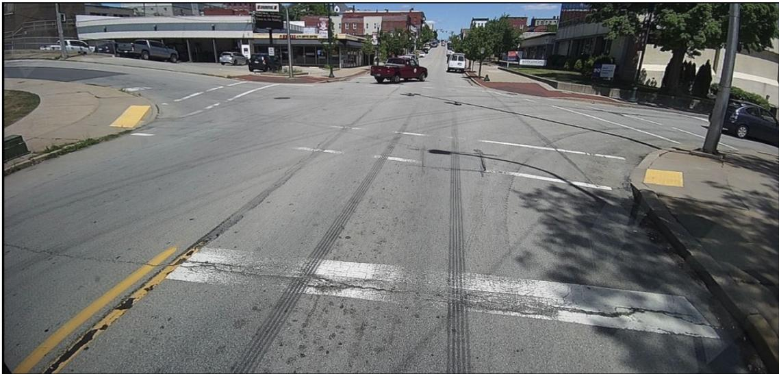
Figure 5.28: An example of where paint from a plain crosswalk has eroded over time, presenting a challenge for object detectors.
