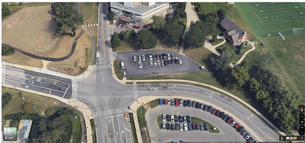
(b) Aerial image of intersection (source: Google Maps accessed 06/10/2023)
