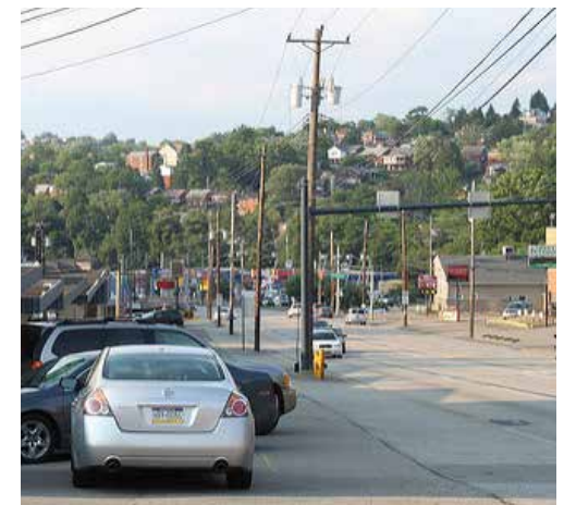
Figure 41 | Auto-oriented corridors without multimodal facilities and street trees are often not visually attractive or friendly environments.
