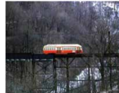
Mckinley Bridge at Bausman Street, wood replaced with steel structure 1929
