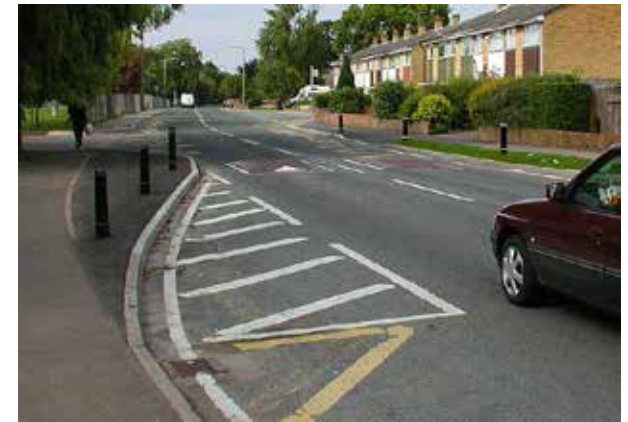
Figure 16 | Bump-outs help to slow traffic and reduce the roadway width for pedestrian crossing safety.
