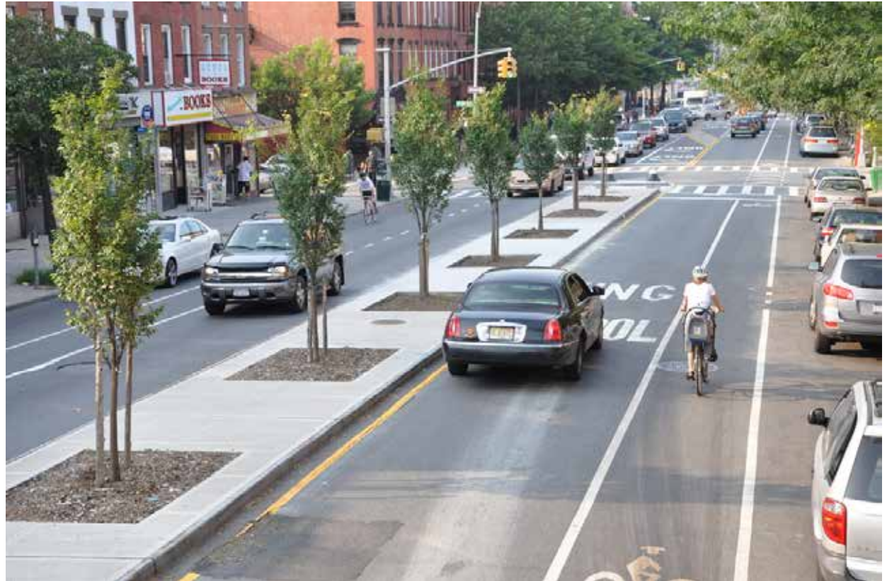
Figure 49 | Converting existing four-lane corridors into complete streets provides a safer condition for all users of the corridor. Street trees provide perceptual enclosure to the right-of-way, naturally slowing vehicle speeds.
