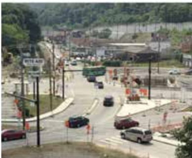
Construction at Route 88 Intersection 2015
