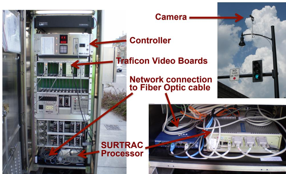
**Figure 2: SURTRAC Hardware Configuration at an intersection**
