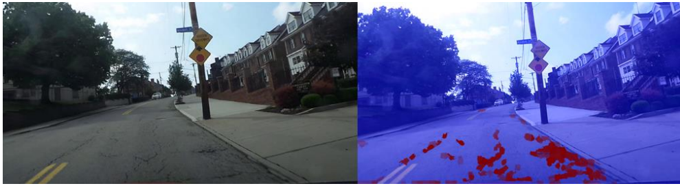
Figure 2 Left: A typical road image. Right: Classification result. The color indicates the severity of distress: blue = no cracks, light to dark red = light to severe cracks.
