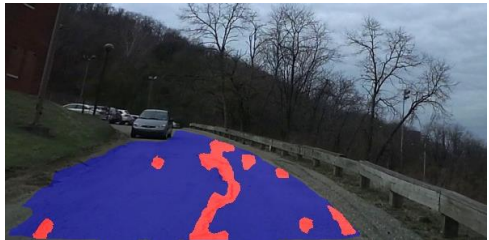
Detection of cracks
